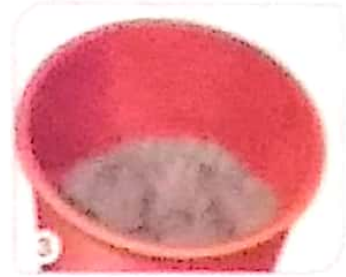
3 Allow the resultant wet mortar to stand for 5 mins for the additive to dissolve. Use the mix within 20-30 mins for best results.
