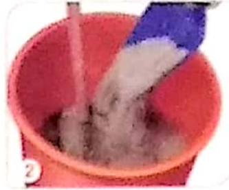
2 In 10 - 12 l of water, add 40kgs of Birla Aerocon Block Jointing Mortar. Stir mix continuously for 5 - 10 mins by using electric mixer or by hand to obtain homogeneous lump-free mix.
